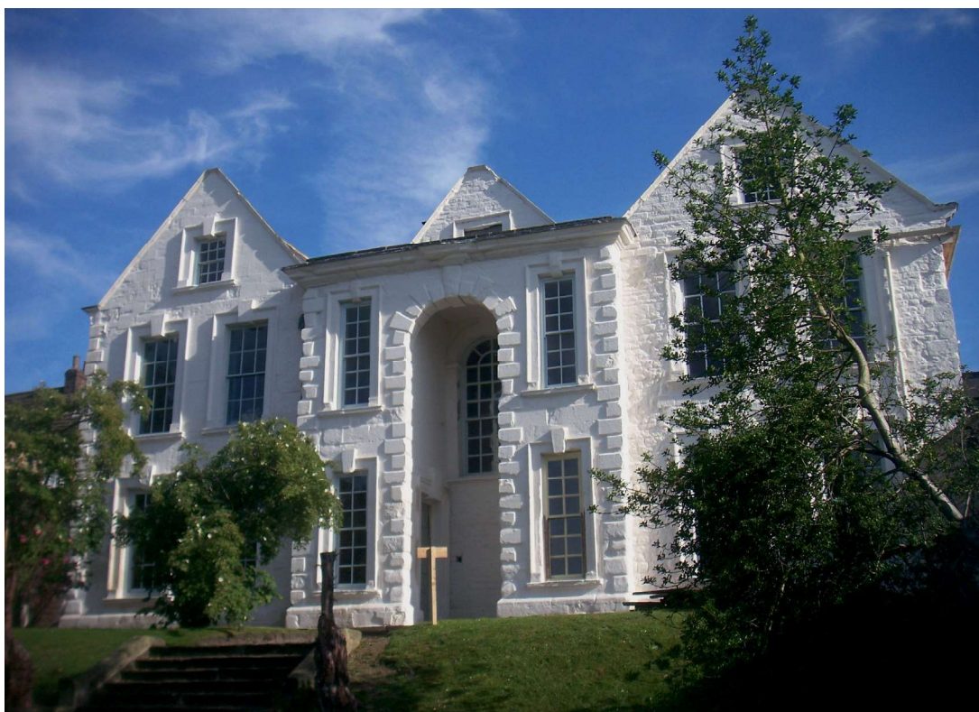
Fig. 2 York House, Malton: aggregated limewash and shelter coat, hot-mixed and applied while still warm.
