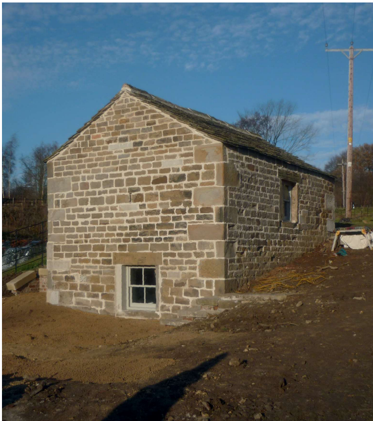
Fig. 10 Hot-mixed lime and sand mortar, Dam Head Pumphouse, Bretton Park, Yorkshire Sculpture Park.
