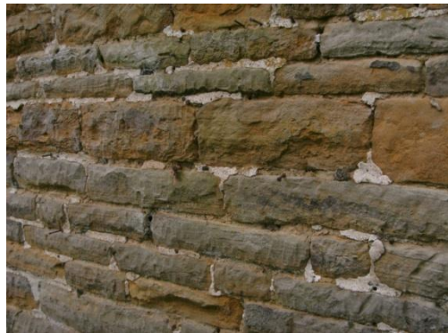
Figure 4 : Pond Farmhouse, Crambe, earth mortar, hot-mixed, haired lime pointed. A Cruck house from circa 1580
