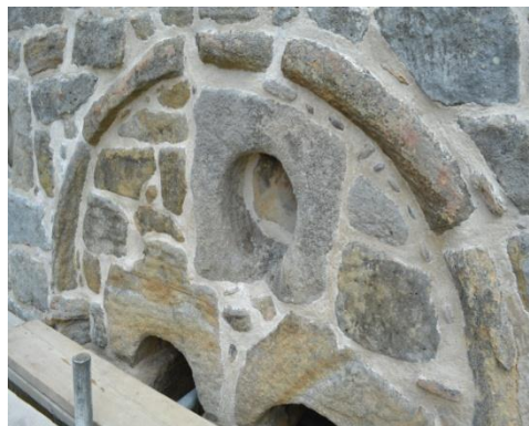
Figure 8. St Andrews, Bywell detail. Mortar 6 quicklime: 20 sand before mixing; afterwards 13: 20
