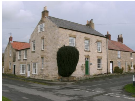
Figure 3: Prospect House, Slingsby. Pointed with hot-mix 2008. Stone geology the same as opc-pointed buildings to either side, but fabric now so dried out that this would not be assumed at first glance.
