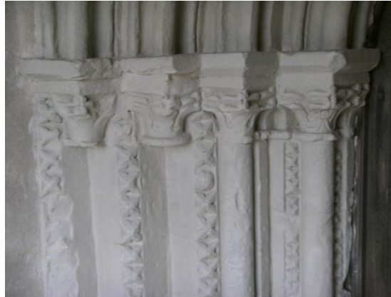
Figure 7 : Hot-lime sheltercoat to Hildenley limestone Early English Doorway, Bossall, near York
