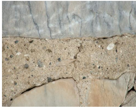
Figure 1 : West Rutland, Vermont, USA; lime lumps indicators of hot-mixing.
