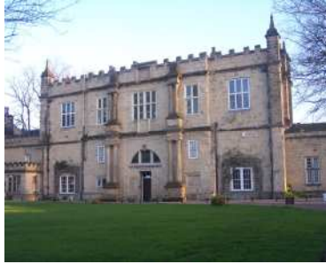
Figure 2: subsequently extended 1604 gatehouse of Eure mansion, Malton, constructed using calcareous sandstone, earth mortars and plasters
