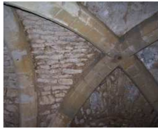
Figures 6 & 7: cross vault with earth mortared walls and lime mortared vault; 12thC ribbed vault with lime mortared ribs and earth mortared fill illustrating informed and deliberate mortar selections by stonemasons
