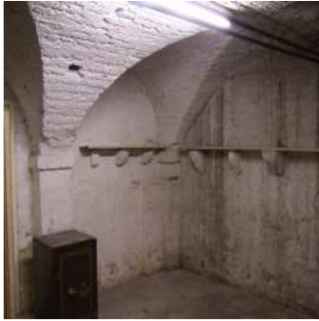
Figures 6 & 7: cross vault with earth mortared walls and lime mortared vault; 12thC ribbed vault with lime mortared ribs and earth mortared fill illustrating informed and deliberate mortar selections by stonemasons
