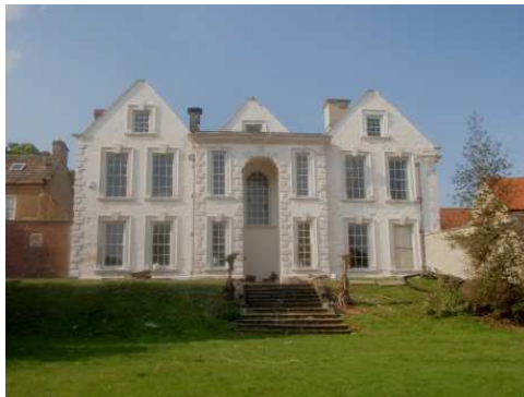
Figure 3: S elevation, York House, Malton. Central range and windows introduced around 1690, using earth and 5% quicklime mortars and hay-rich earth plasters with limestone dust, quicklime and oxhair finish coats over.
