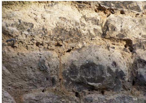
Figure 10 mud-mortared limestone, Malton
